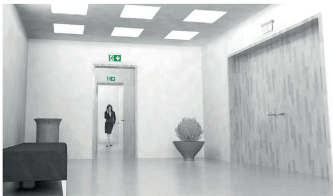
During normal operation, the pathfinder luminaire indicates the designated 1st escape route. Indication of the alternative 2nd escape route is not visible.
